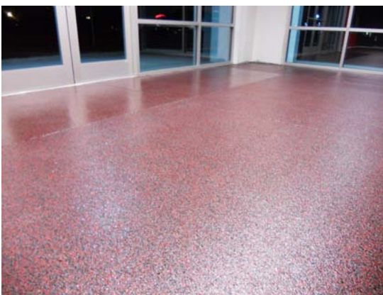
One topcoat in front, two in back - 1/4" color chips
